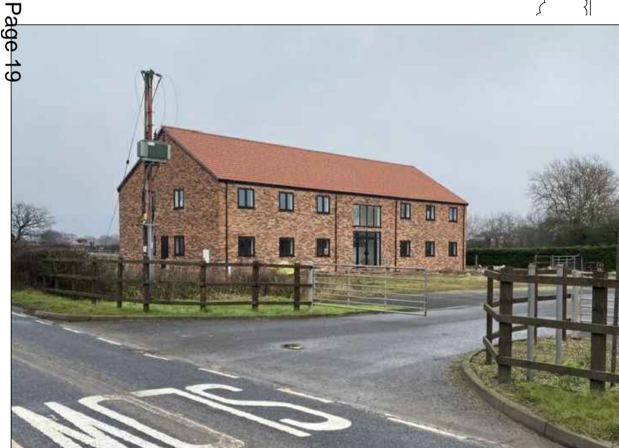
Medvance House, Burn (between ring road and Common Lane) Example of 'business expansion' Selby in open countryside Ref 2015/1210/FUL
