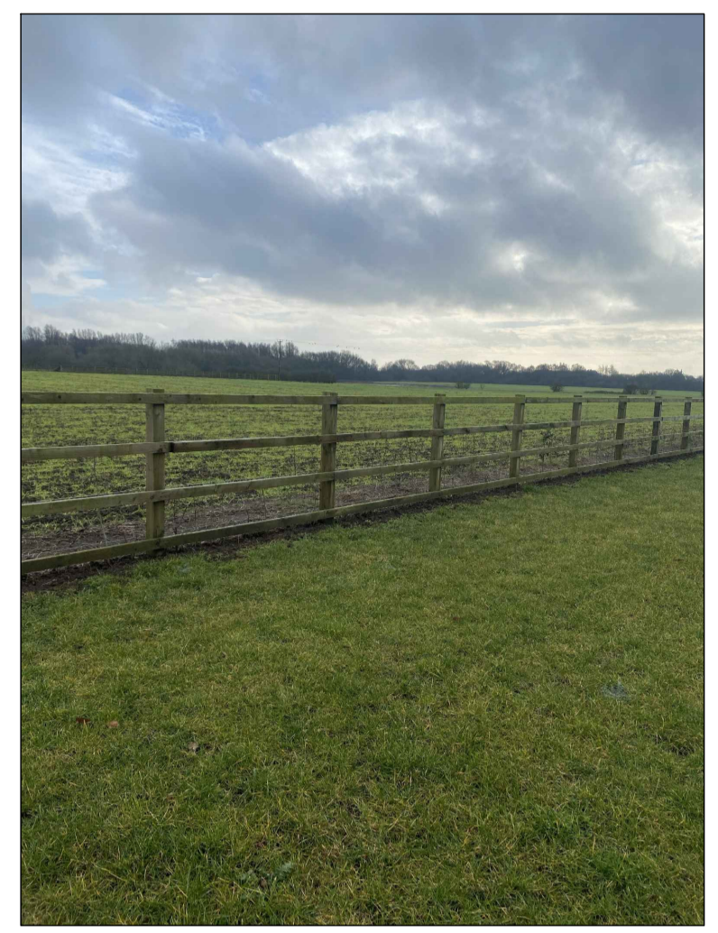
1.2m High post and rail fence
